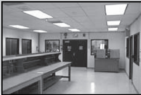
Test enclosure for hazardous machinery device evaluation. Controls and monitors to regulate the test environment as well as both wet and dry fire suppression are installed.
