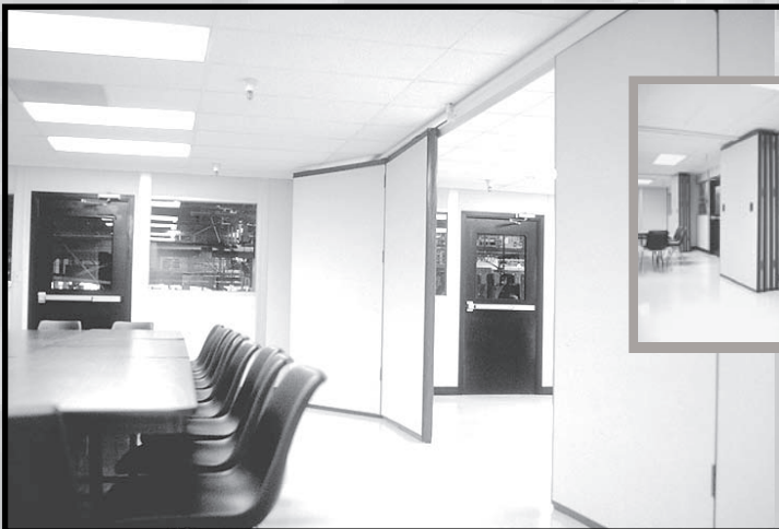
Training rooms located adjacent to an automobile assembly area provide acoustical privacy. Operable acoustical walls quickly divide larger areas into smaller meeting rooms.
