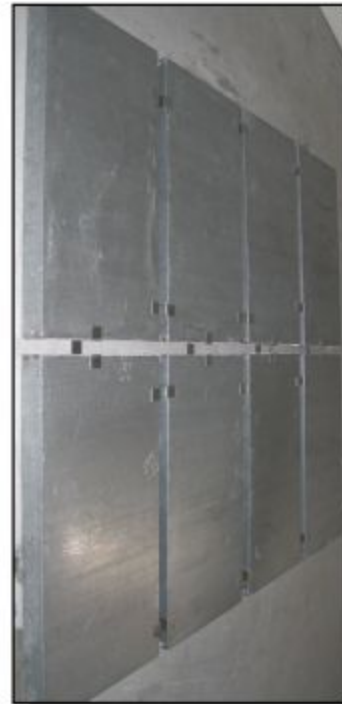
Type SF Absorptive Panels Installed On Concrete Wall
